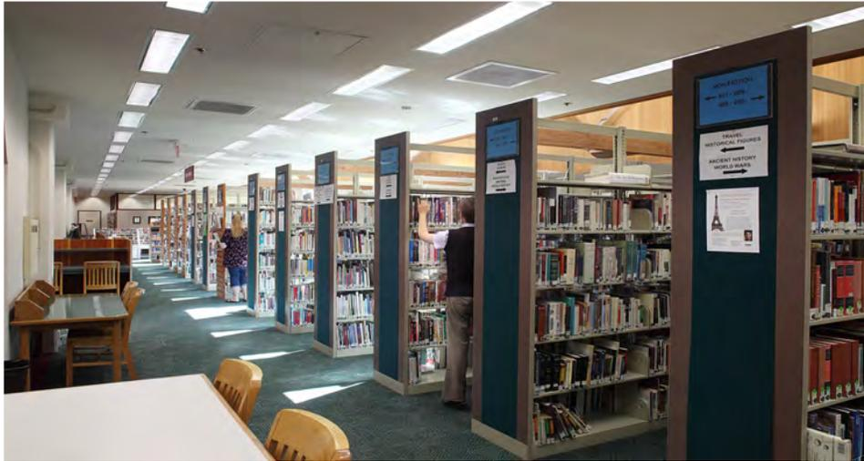
◀ The lighting control system adjusts light levels and corresponding energy usage based on occupancy. In unoccupied areas (shown in the foreground), light levels are dimmed. When someone walks into the space (shown near the 3rd bookcase) occupancy sensors sense their arrival and light levels increase to full output.
