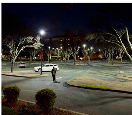
◀ When occupancy sensors sense the approach of a pedestrian or car, the bi-level LED fixtures adjust from low light levels (on the left) to high light levels (on the right).
