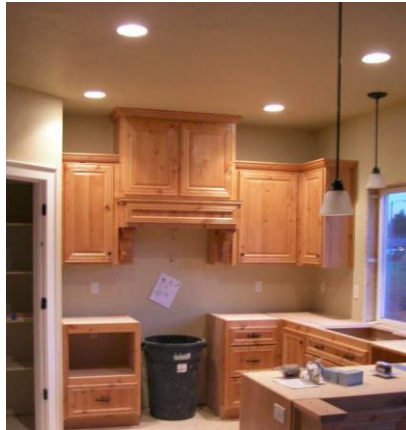
FIGURE 11. LED DOWNLIGHT FIXTURE AND RESIDENTIAL INSTALLATION EXAMPLE (DOE GATEWAY DEMONSTRATION)
