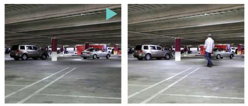
▲ Bi-level light fixtures utilize occupancy sensors to reduce light levels when the space around the fixture is unoccupied (image on left). When someone walks into the space, light fixtures automatically switch to 100% light output (image on right). This automated lowering and elevating of light levels depending on occupancy saves energy and increases fixture life.
